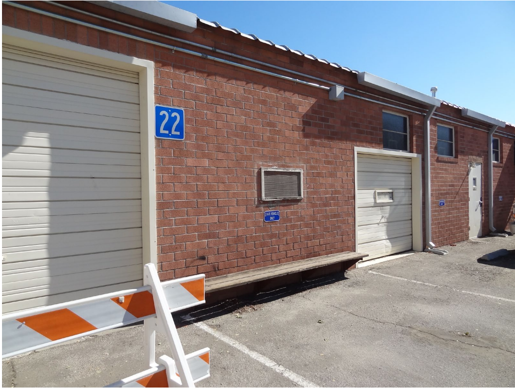
Maintenance / Housekeeping – Building #22 – FCA Building #0353 Description: Exterior of the Building.
