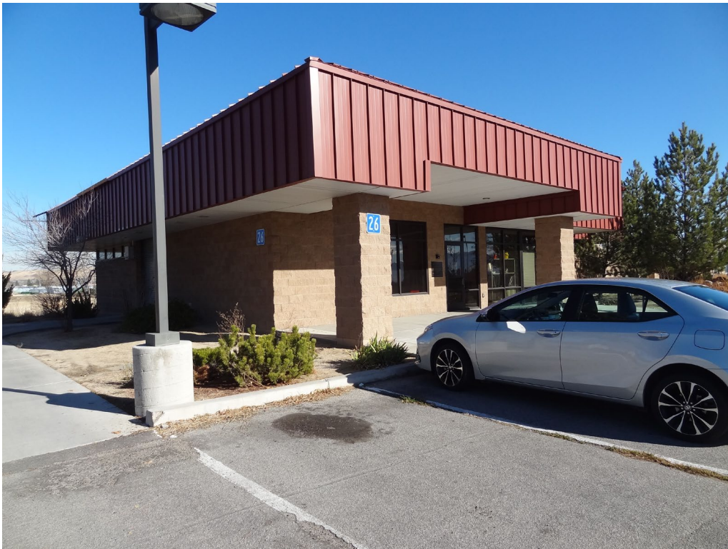
Central Kitchen – Building #26 – FCA Building #2725 Description: Exterior of the Building.
