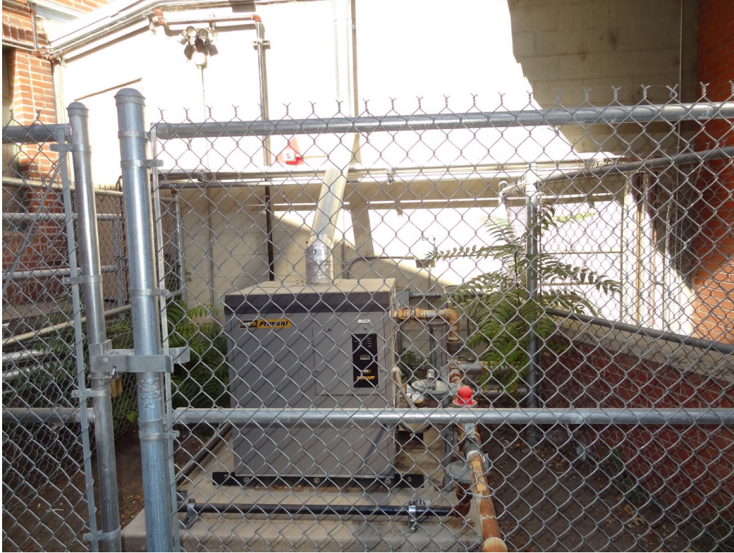
Medication Clinic – Building #5 – FCA Building #0352 Description: Boiler Replacement.
