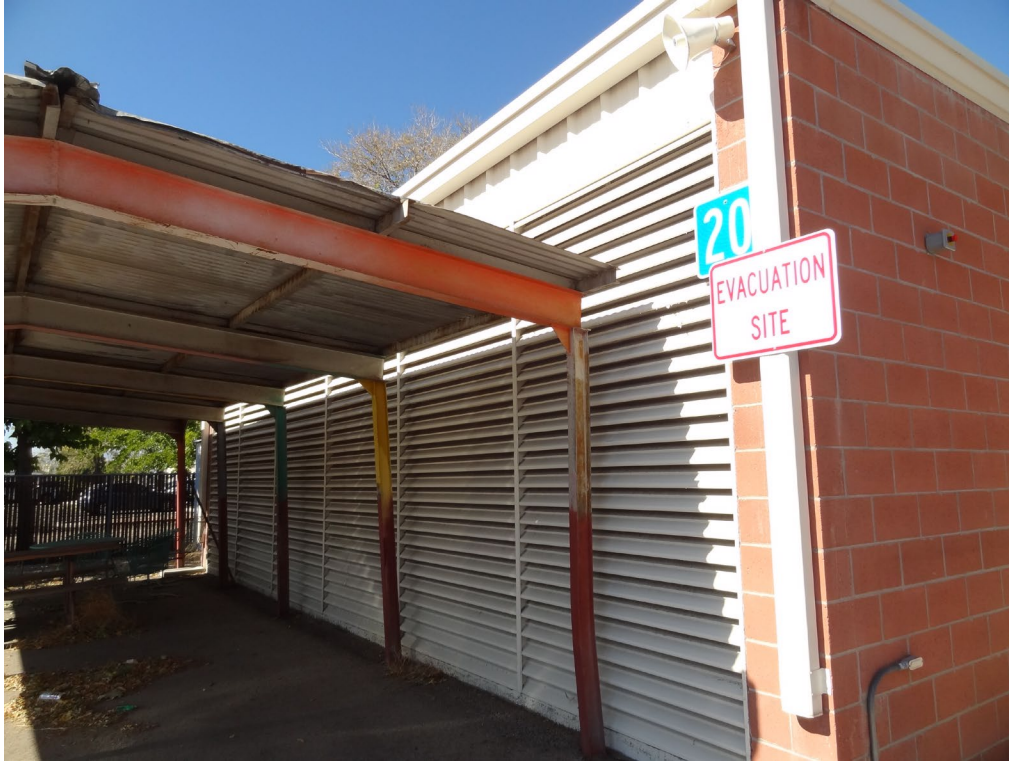
Generator Building – Building #20 – FCA Building #0347 Description: Exterior of the Building.
