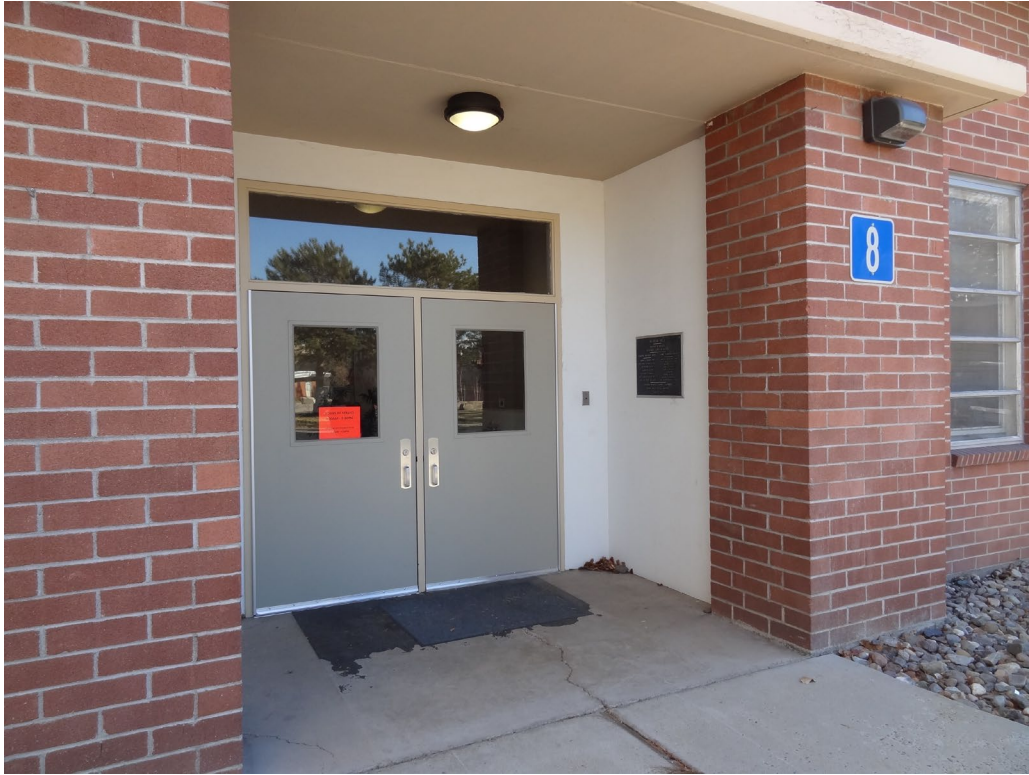
Building #8 – FCA Building #0340 Description: Exterior of the Main Entry.
