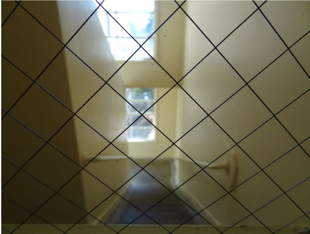
Administration – Building #1 – FCA Building #0326 Description: Interior Stair Handrail Replacement.
