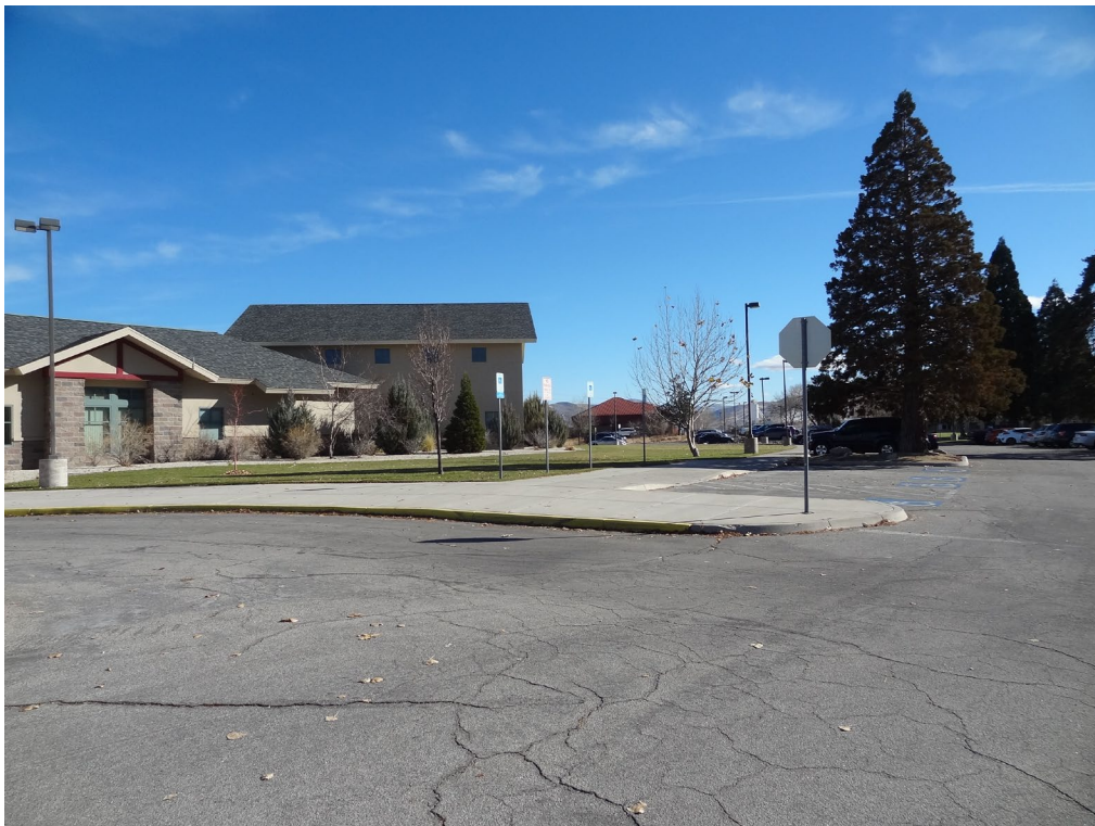
Dini-Townsend Hospital – Building #25 – FCA Building #2449 Description: Exterior of the Building.
