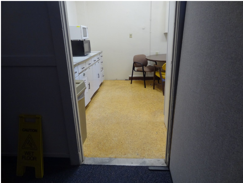
Administration – Building #1 – FCA Building #0326 Description: Break Room Remodel.
