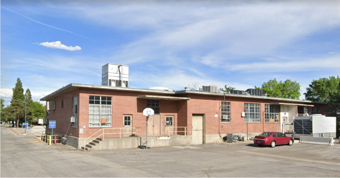
Building #10 – FCA Building #0339 Description: Demolish Structure Recommendation.
