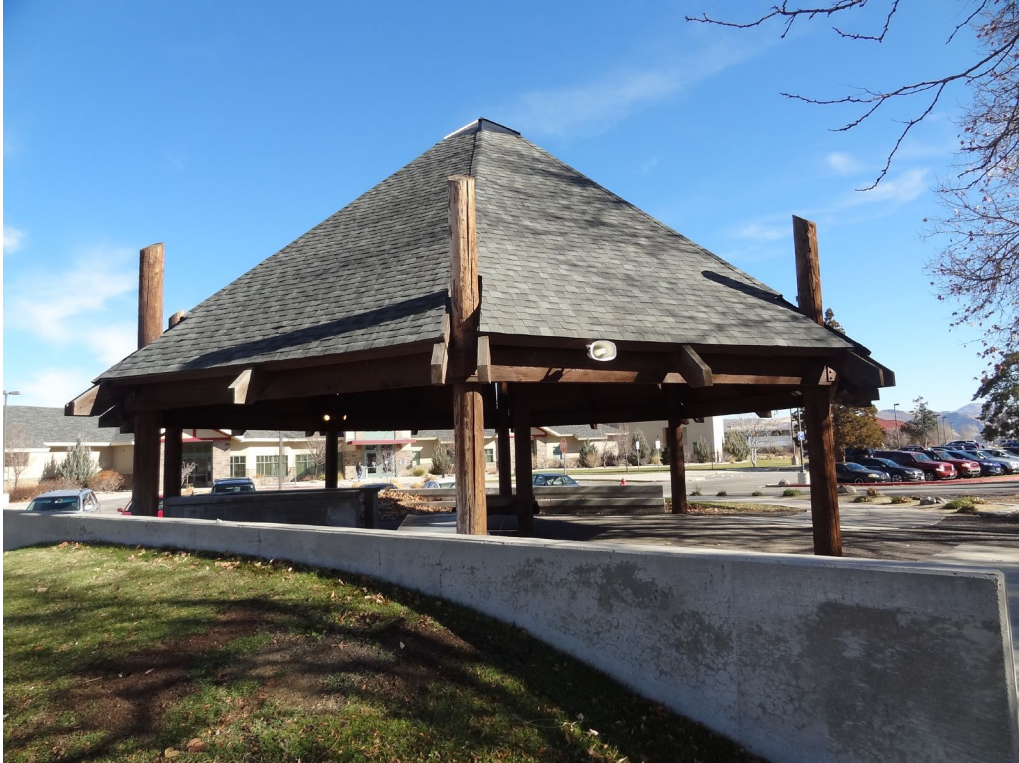
Gazebo – FCA Building #0976 Description: Exterior of the Structure.
