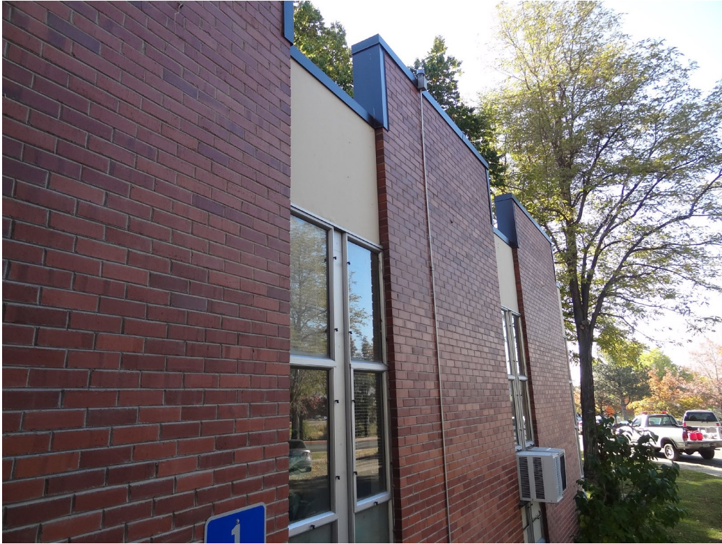
Administration – Building #1 – FCA Building #0326 Description: Exterior of the building.
