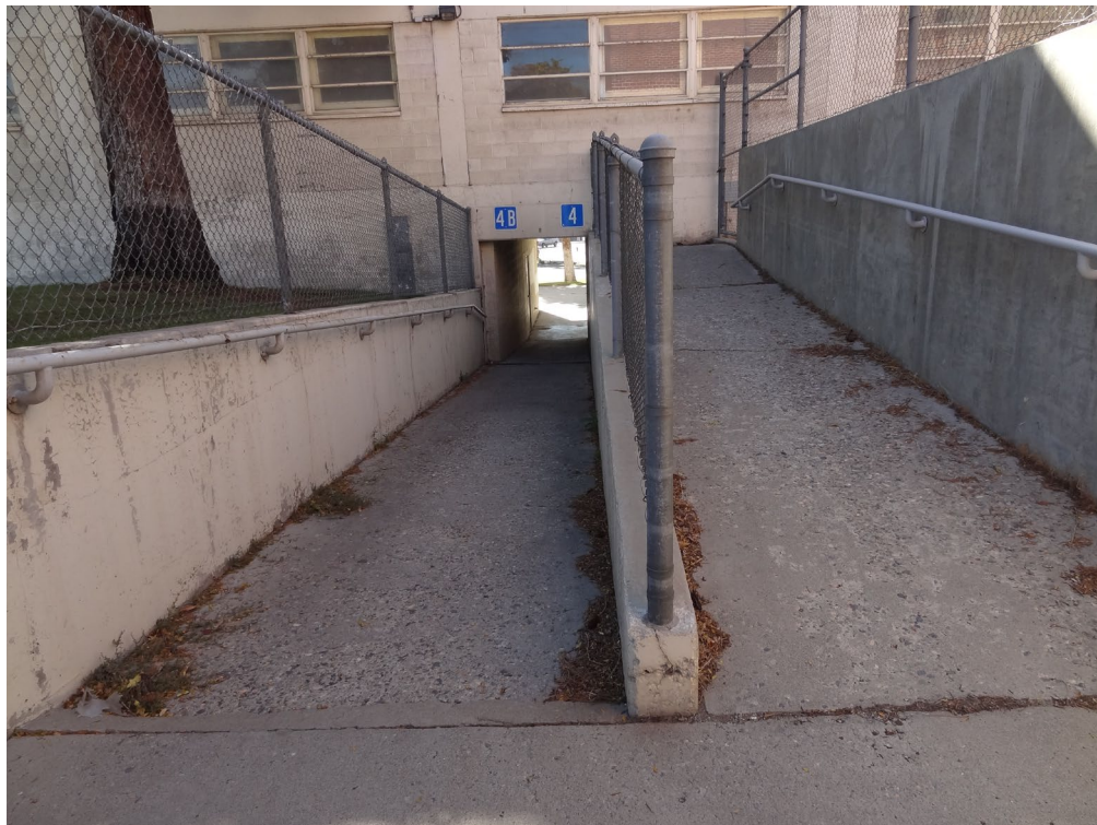
Building #4 (Vacant) – FCA Building #0329 Description: Demolish Structure Recommendation.
