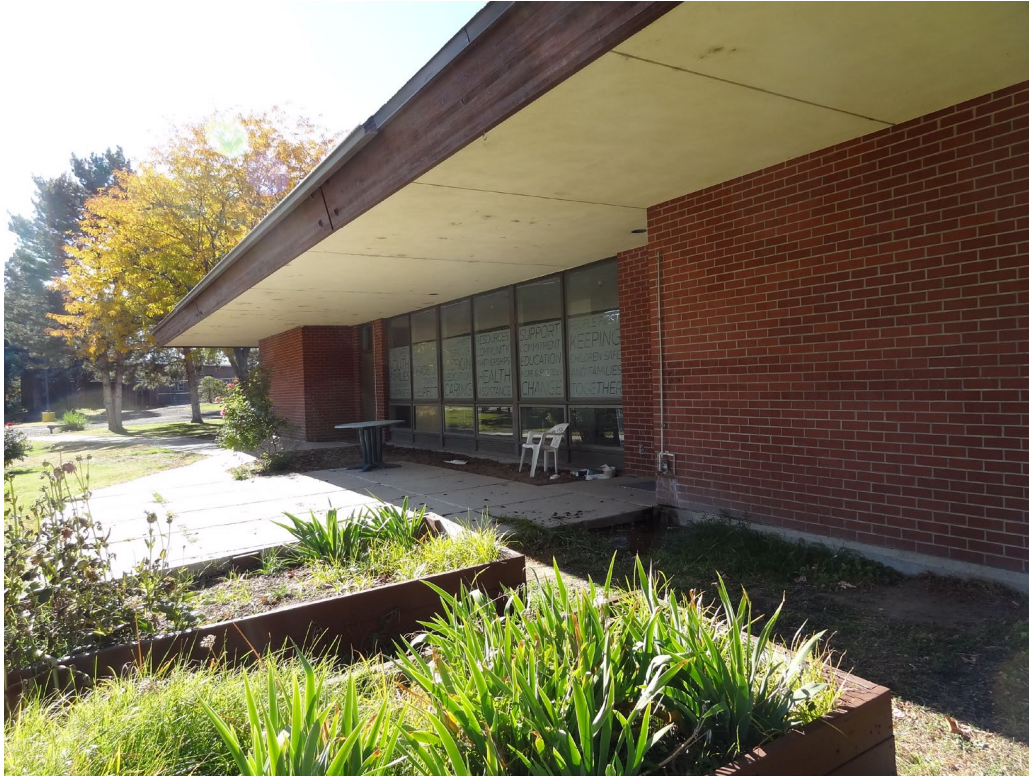
Group Home – Building #8B – FCA Building #0333 Description: Exterior of the Building.
