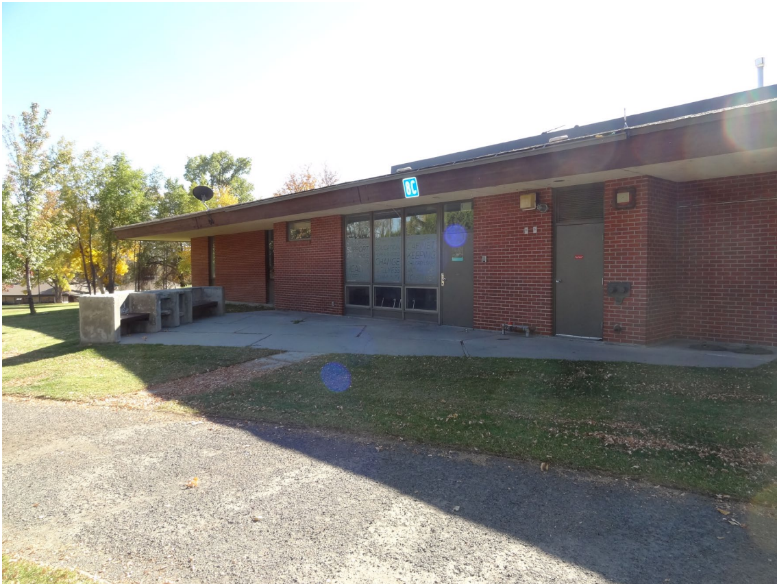
Group Home – Building #8C – FCA Building #0334 Description: Exterior of the Building.
