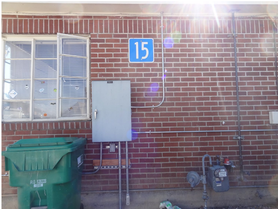
Group Home – Building #15 – FCA Building #0343 Description: Exterior of the Building & Window Replacement.
