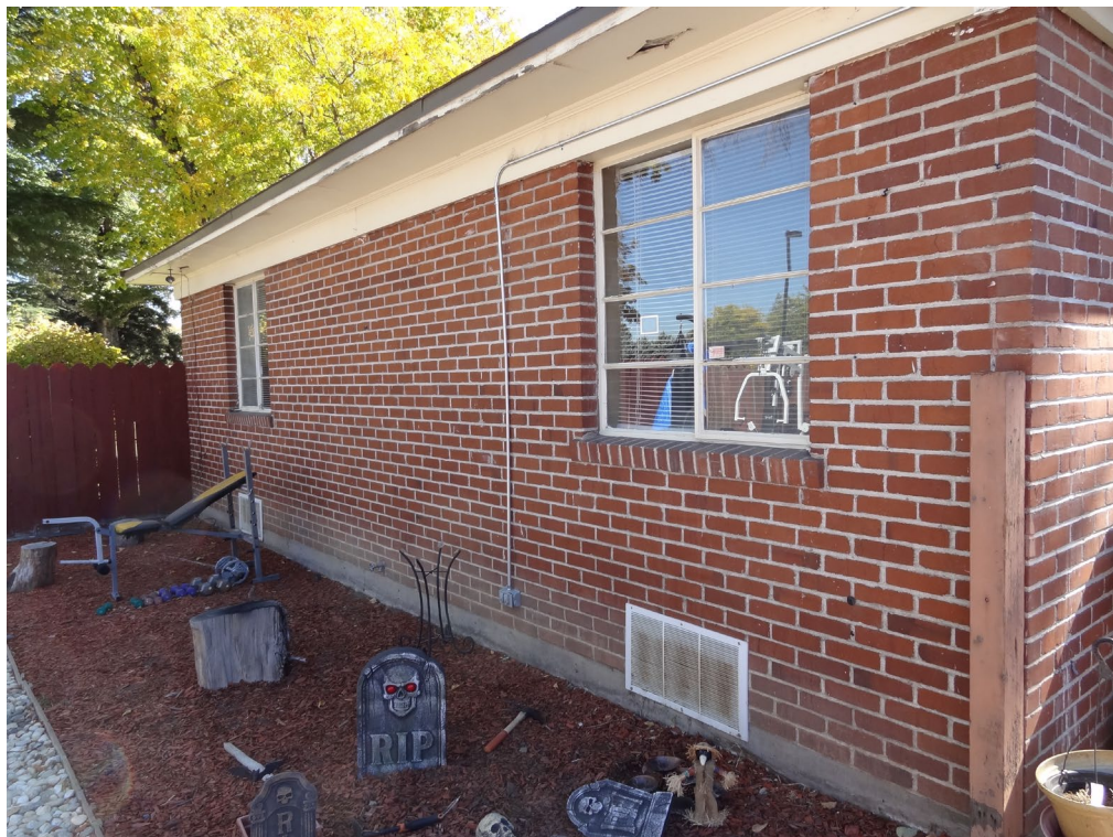
Group Home – Building #14 – FCA Building #1958 Description: Exterior of the Building.
