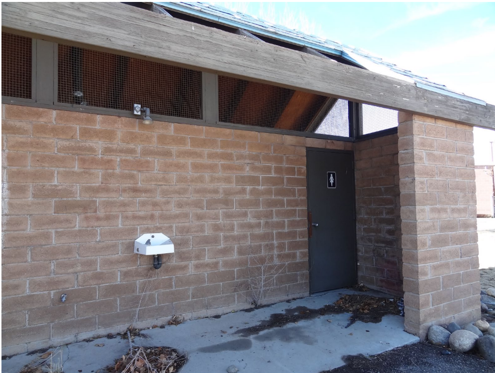
Gazebo Restroom – Building #27 – FCA Building #0521 Description: Demolish Structure Recommendation.
