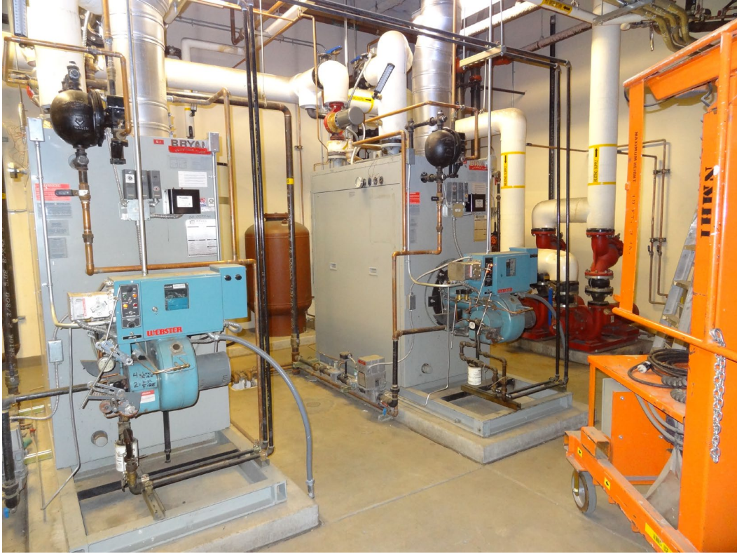
Dini-Townsend Hospital – Building #25 – FCA Building #2449 Description: Mechanical Room.
