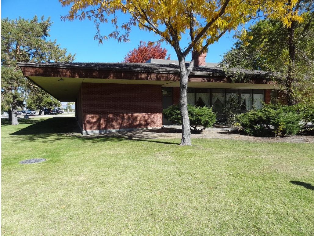
Group Home – Building #8A – FCA Building #0330 Description: Exterior of the building.
