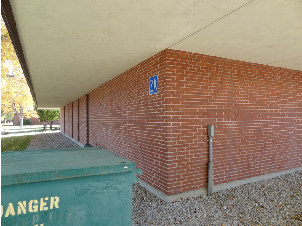
Library / Meeting Rooms – Building #2A – FCA Building #0328 Description: Exterior Finishes of the Building.
