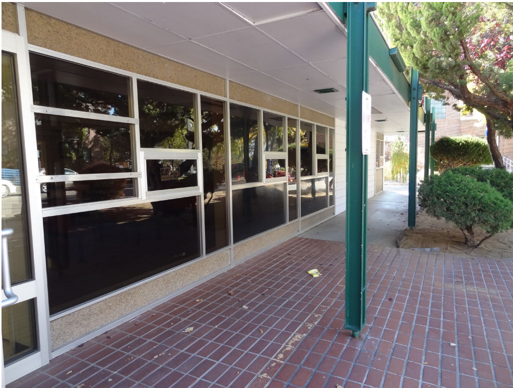
Canteen – Drop In Center – Building #2 – FCA Building #0327 Description: Exterior of the Building.
