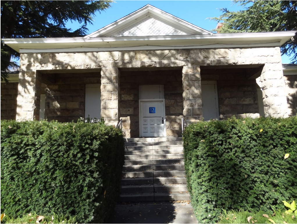
Building #12 – Historical (Vacant) – FCA Building #2059 Description: Exterior of the Building.
