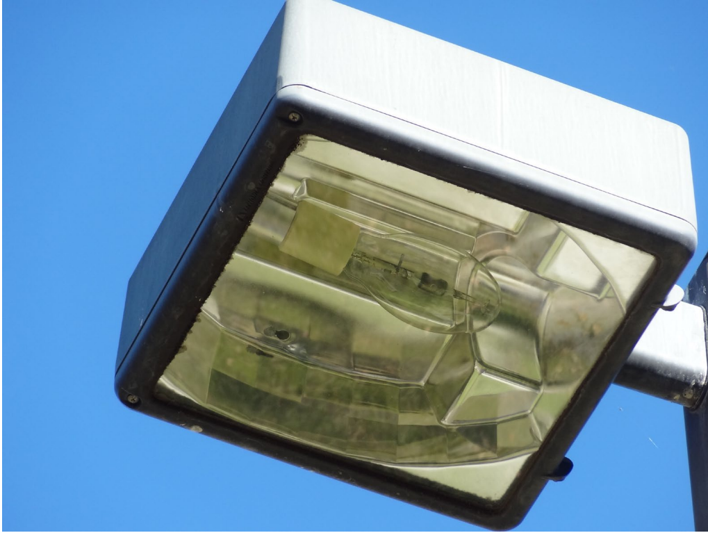
Northern Nevada Adult Mental Health Services Site – FCA Site #9985 Description: Sitewide Exterior Lighting Upgrades.
