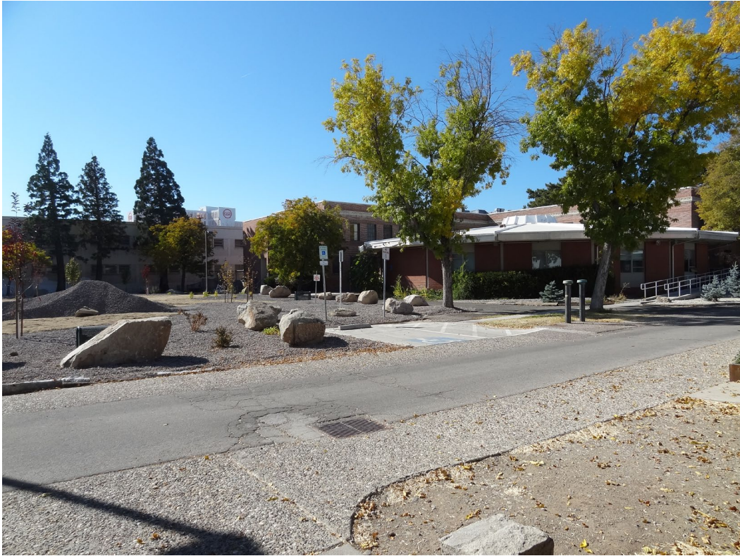
Northern Nevada Adult Mental Health Services Site – FCA Site #9985 Description: Concrete & Paving Upgrade Sitewide.
