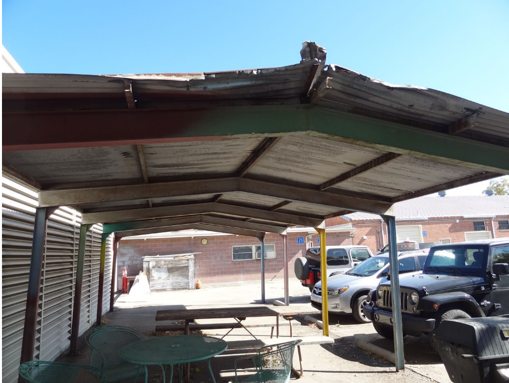
Parking / Shade Ramada – FCA Building #2677 Description: View of the Building.
