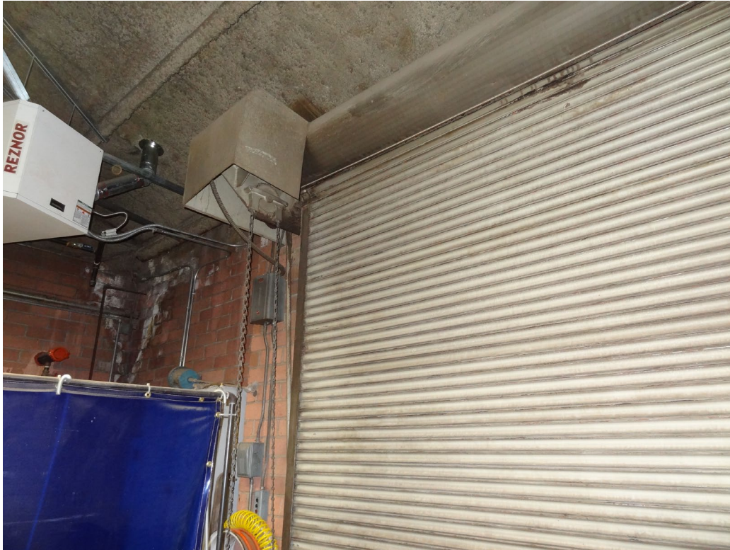
Maintenance / Housekeeping – Building #22 – FCA Building #0353 Description: Overhead Door Replacement.
