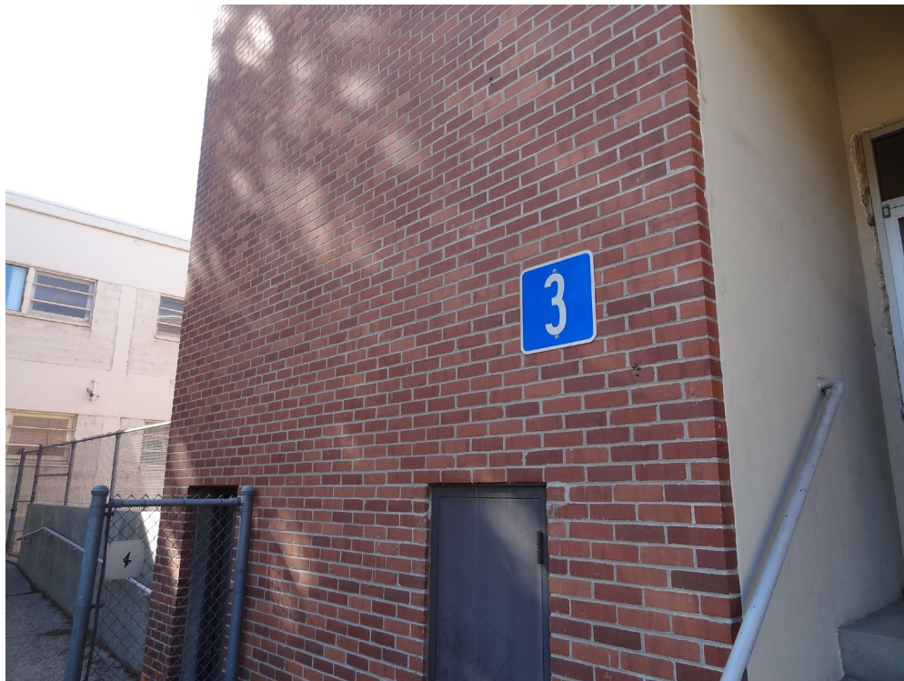
Lab / Pharmacy – Building #3 – FCA Building #0331 Description: Exterior of the Building.
