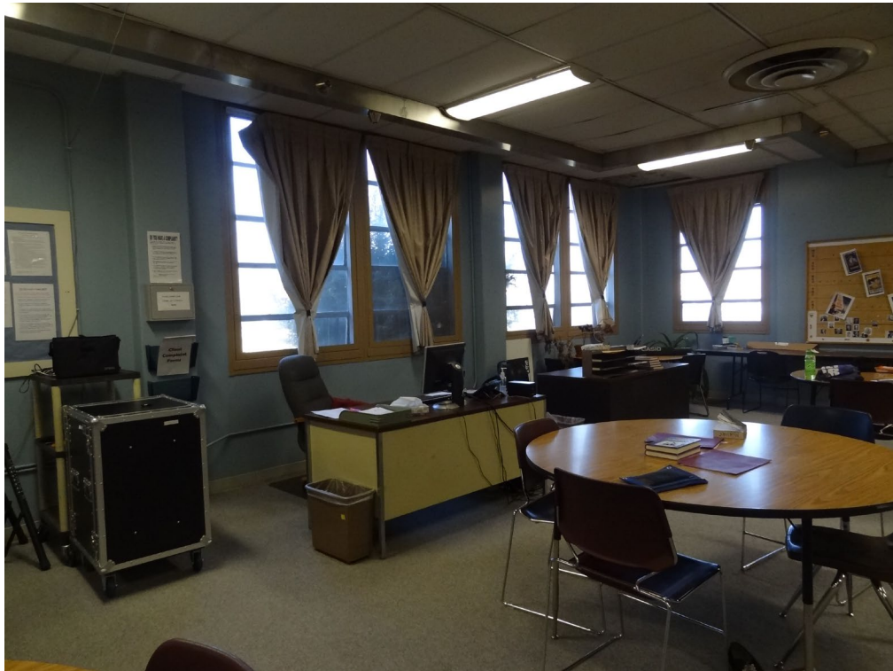
Building #8 – FCA Building #0340 Description: Window Replacement.
