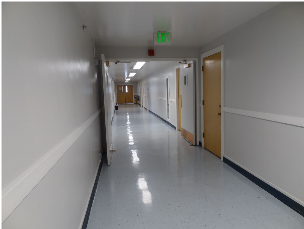
Administration – Building #1 – FCA Building #0326 Description: Lever Hardware Installation.
